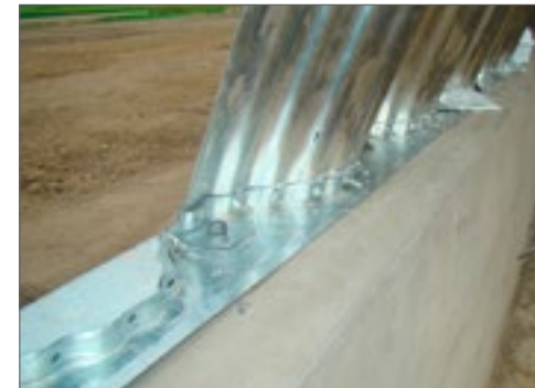
ARCHWALL 4500 FOOTING CHANNEL
