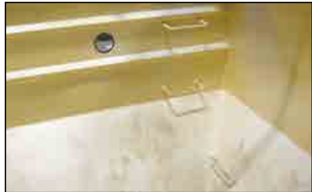
Fig 21 - Compartment ladder rungs
