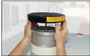
Fig 9 - Inspect vents for correct operation
