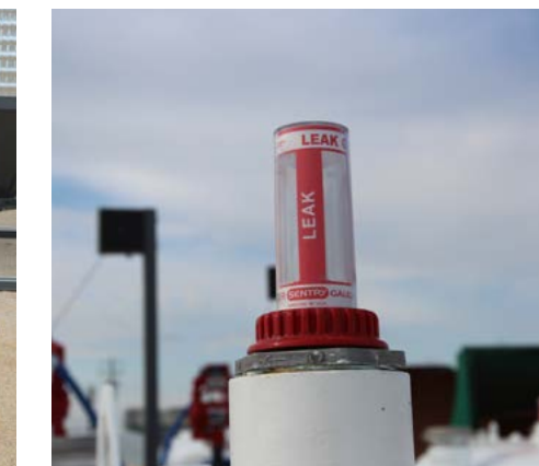
LEAK DETECTION GAUGE
