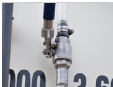
Liquid Site Gauge Valve Safety enclosure for added security.
