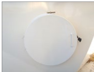
Roof Manhole Access hole in top cone.
