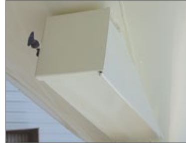
Poke Hole 8" x 8" access to discharge just above gate.
