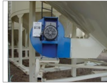
Fan Mounting Bracket Support bracket mounted under fan.
