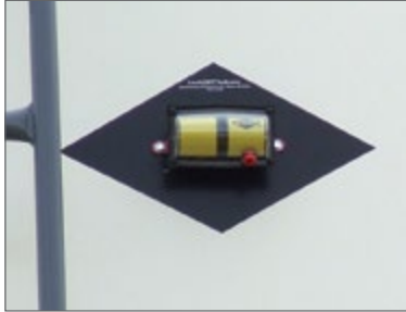
LevAlert Level indicator on sidewall.
