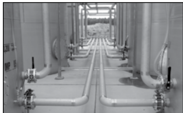
Fig 22 - Fill and discharge tubes
