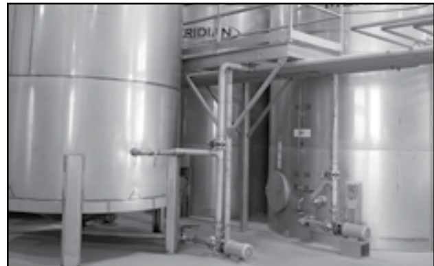
Fig 20 - Permanent fill and discharge system
