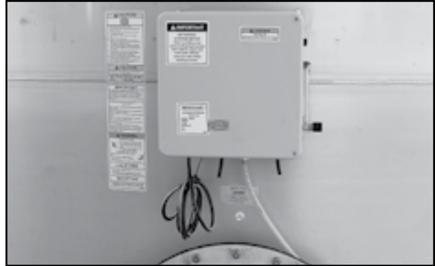
Fig 13 - Airmix liquid fluidizer control box
