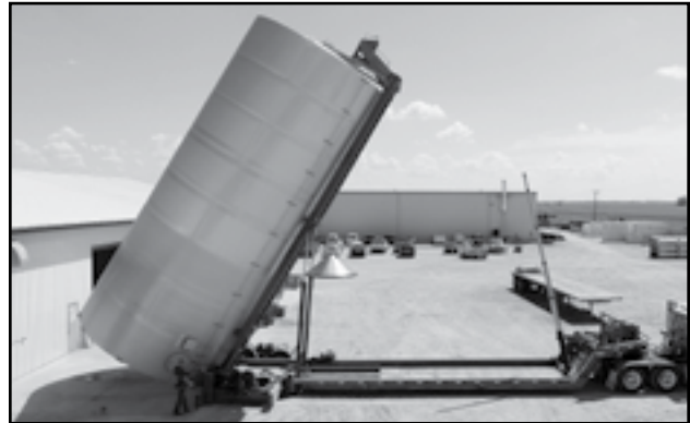
Fig 4 - Unloading tank
