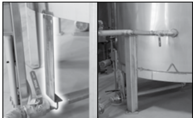
Fig 8 - Bracket to support piping from bottom coupler
