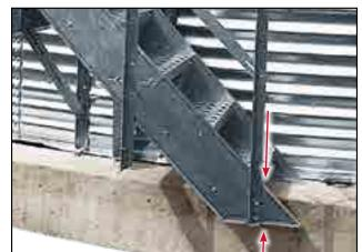
Fig 20 - Remove tripping hazard
