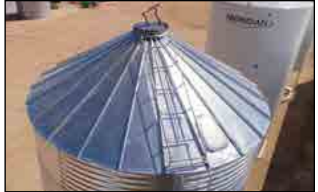
Fig 7 - SC Roof ladder
