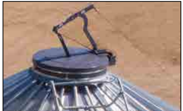
Fig 9 - Loading hatch covered by the lid
