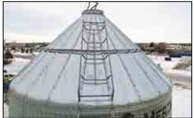
Fig 8 - DC Roof ladder
