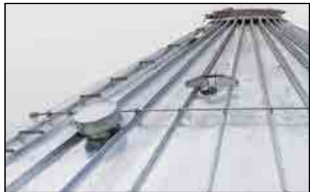
Fig 16 - Roof vents and stiffeners
