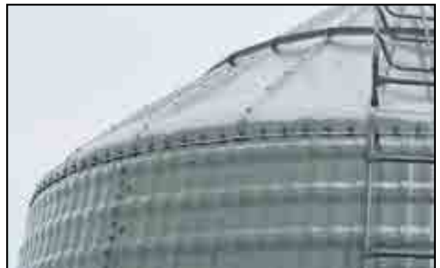
Fig 10 - Sealed roof eave
