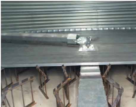
Welded truss support
