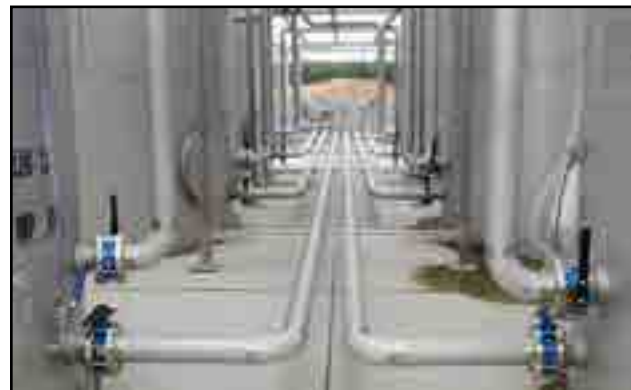
Fig 22 - Fill and discharge tubes
