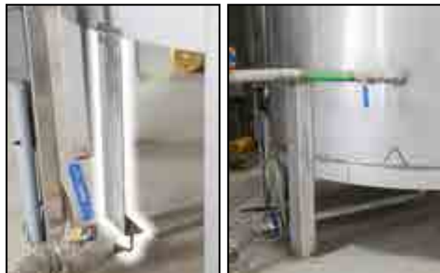
Fig 8 - Bracket to support piping from bottom coupler
