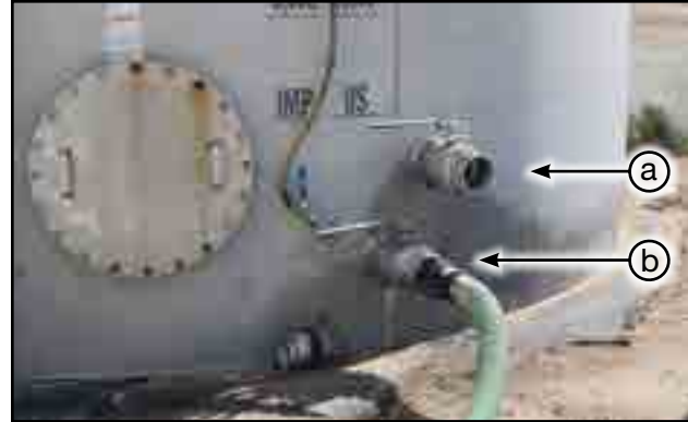
Fig 19 - Fill (a) and discharge (b) couplers
