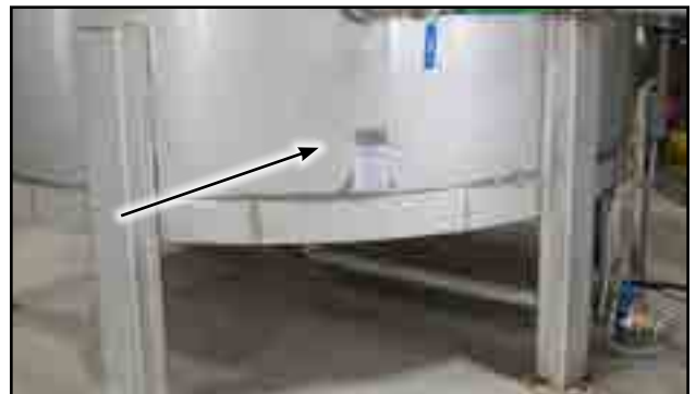
Fig 1 - Serial number location on chemical tank
