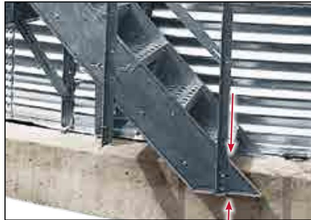
Fig 20 - Remove tripping hazard
