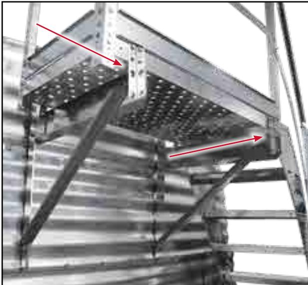
Fig 9 - Short posts on A-frame connected to platform
