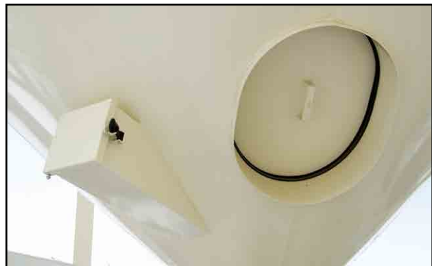
Fig 12 - Poke Hole and bottom manway
