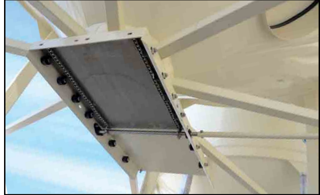
Fig 4 - Slide gate attached below unloading chute
