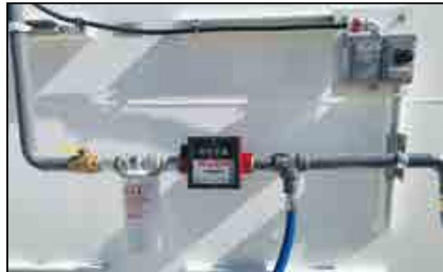
Fig 24 - Pump filter and meter
