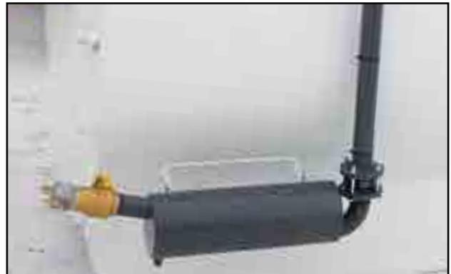
Fig 17 - Bottom fill tube with cam lock
