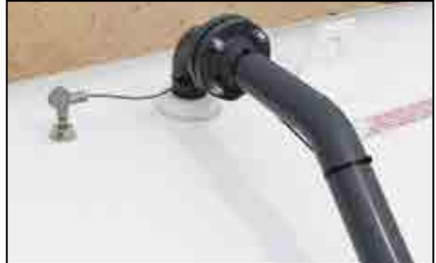
Fig 16 - MECO Overfill Alarm is connected to the fill tube
