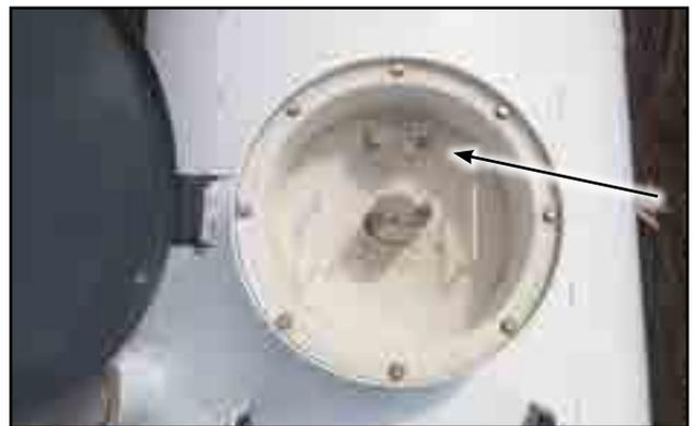
Fig 22 - Inside Spill Box is the Dip Port
