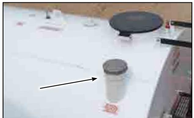
Fig 11 - Secondary containment emergency vent
