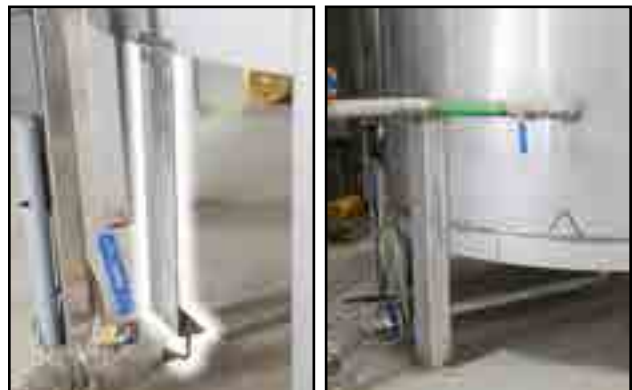
Fig 8 - Bracket to support piping from bottom coupler
