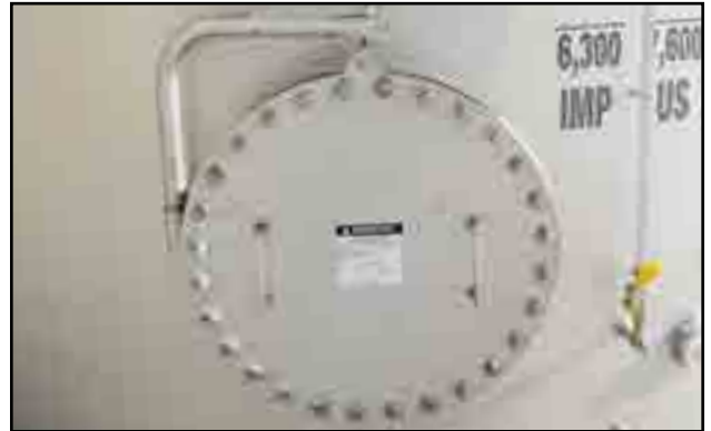
Fig 25 - Manway on flat bottom tank
