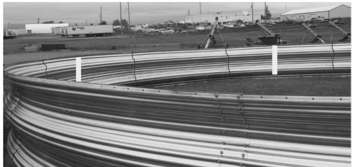
8. Once all struts are installed, install the remainder of the bolts on every panel joint. Overlap second Ring Panels to the outside of the first ring. The second ring of panels must be placed on the outside of the first ring to prevent water from entering the grain ring. The seam lines for the second ring must be offset from those on the first ring by at least 8 bolt holes.
