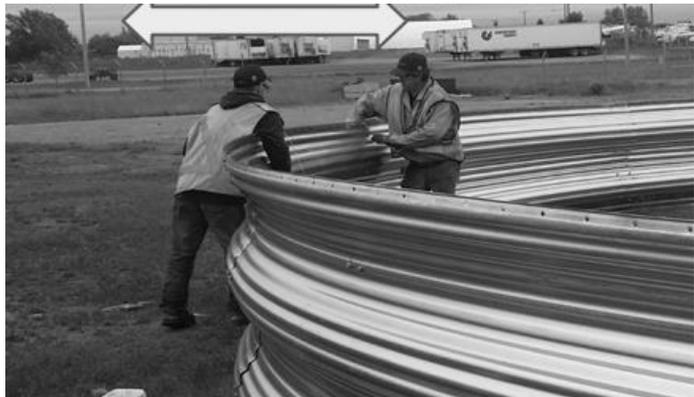
7. Once panel is aligned install strut (there should be a strut every second panel)
