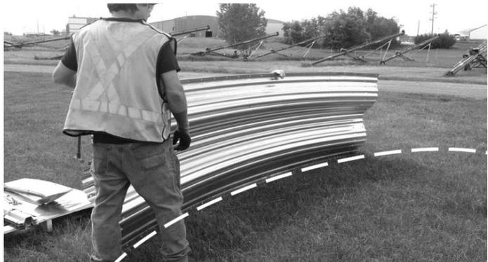
3. Once aligned, drive a strut into the ground (inside circle) and bolt it to 2 humps of panel. Panels must be assembled in a clockwise manner.
