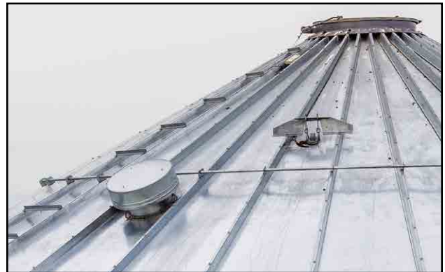
Fig 17 - Roof vents and stiffeners
