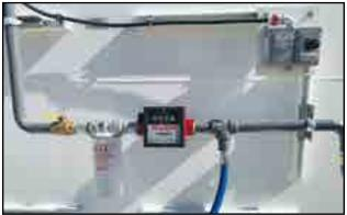
Fig 24 - Pump filter and meter
