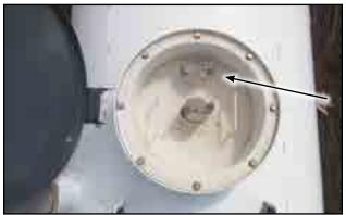
Fig 22 - Inside Spill Box is the Dip Port
