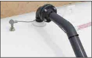
Fig 16 - MECO Overfill Alarm is connected to the fill tube
