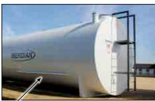
Fig 12 - Dip stick holder and ladder
