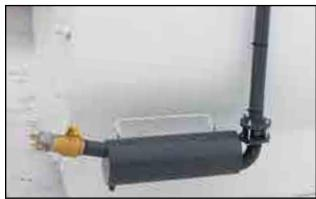
Fig 17 - Bottom fill tube with cam lock
