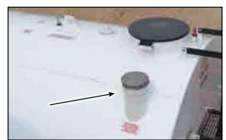
Fig 11 - Secondary containment emergency vent
